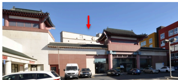
Figure 10: Capitol Milling Company building, view of west elevation from N. Broadway (GPA, 2018)
